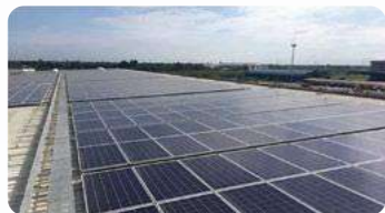
CPALL Convenient Stores and Distribution Center 64 MW, 2,669 Stores 25 DCs, 45,492 tCO 2 e
