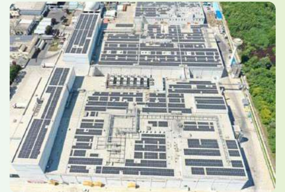
Solar rooftop installation with 5-MW power output Reduced GHG by 90,000 tons CO 2 e
