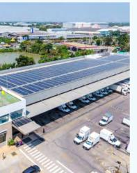
C.P. Group's companies have implemented multiple renewable energy projects, starting with installing solar rooftop electricity generation systems at animal feed factories, food processing factories, distribution centers, office buildings, base stations, and 7-Eleven stores. The solar rooftop system has an installed capacity of 58.9 MWp, and is able to produce over 85 million kWh of electricity per year, which is equivalent to around 49,200 tCO2e of GHG emissions reduction.
